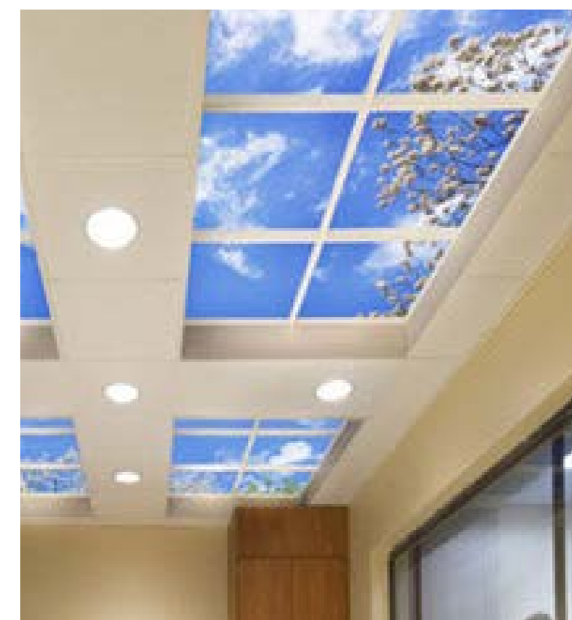
Artificial skylight for visual connection to nature
